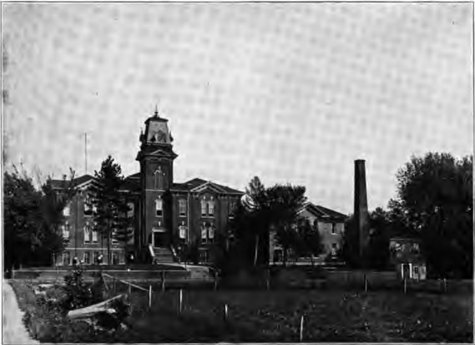
HIGH SCHOOL BUILDINGS, NEVADA
